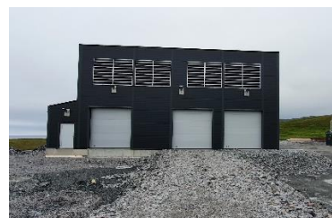
Hydrogenfabrikk i Berlevåg, Varanger KraftHydrogen AS
